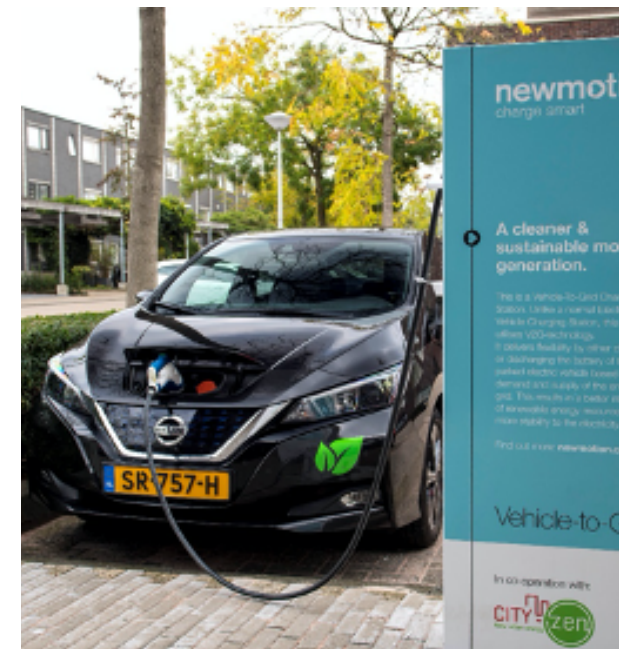
↑ Bidirectional V2G charging station installed for the City-zen VPP pilot. Photo by @ Alliander
